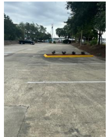
NEW BUSHES IN THE PARKING ISLANDS AT THE ENTRANCE
